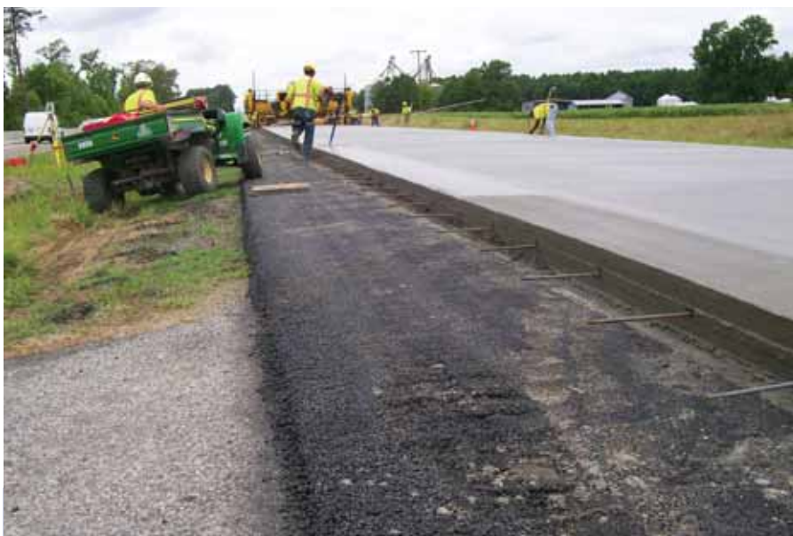
In the unbonded section, they used tie bars to tie the two lanes together and tie the shoulders to the lanes but no reinforcing steel was used.
